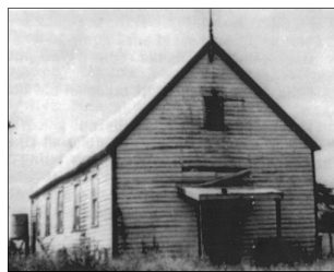
The Hall immediately prior to demolition
