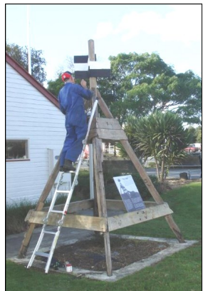
At work on the Trig Station
