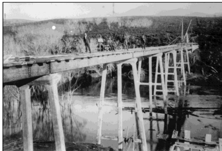
Pukehoua Bridge during construction.
