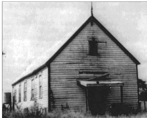
The hall shortly before it was demolished. The wire rope stays appear to have been removed.
