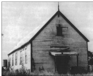
The Hall immediately prior to demolition
