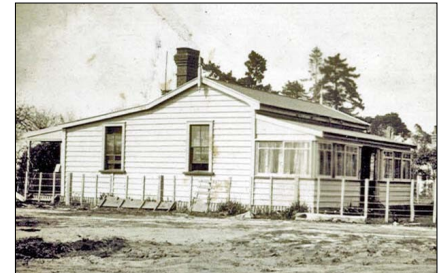
Two rooms were added in the 1930s by enclosing a re-constructed verandah.
