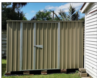
The new storage shed.
