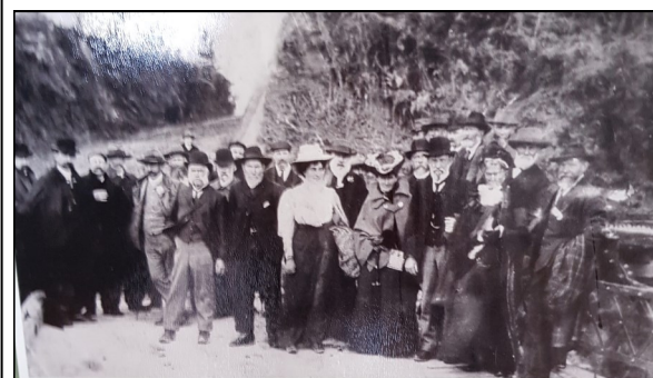
The opening of the Mangapiko (Matakitaki) Bridge October 1905
