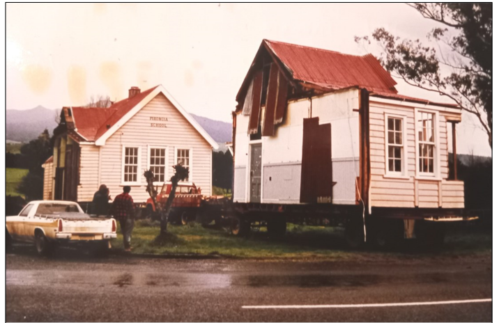
Trucking the building onto the new site in two loads
