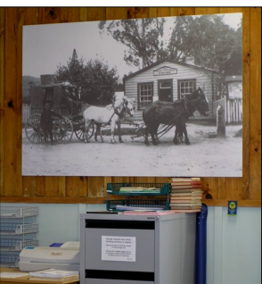
The enlarged picture of the Post & Telegraph Office built in the 1870s.
